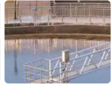
Industrial water storage tank
