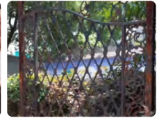
Doors and Windows
